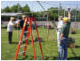
Assembling the VHF Beam
