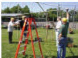
Assembling the VHF Beam
