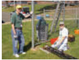
Preparing to Raise the Tower
